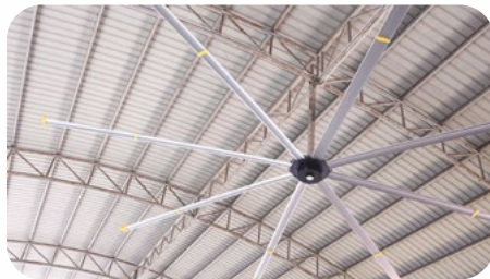
Energy efficient HVLS fans
